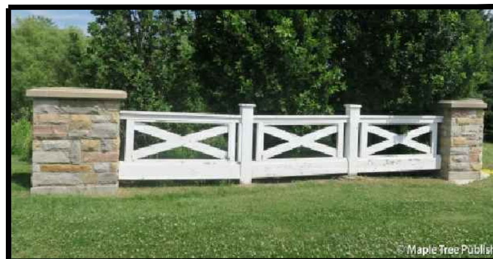
CROSS BUCK FENCE WITH MASONRY "B"
