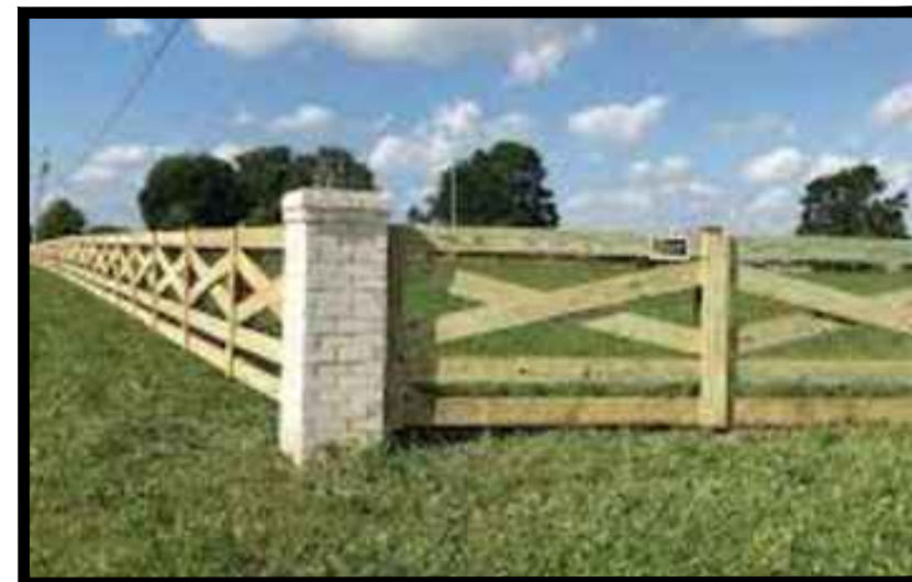
CROSS BUCK FENCE WITH MASONRY "C"
