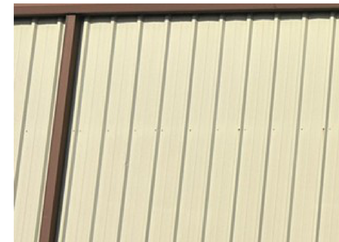
METAL SIDING & TRIM NEW SHOP BUILDING TO MATCH EXIST.
